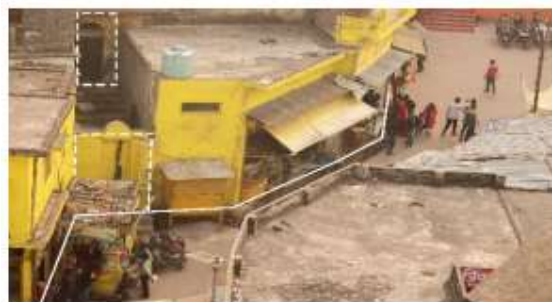
Fig 33: Edge of a street. Source: author
